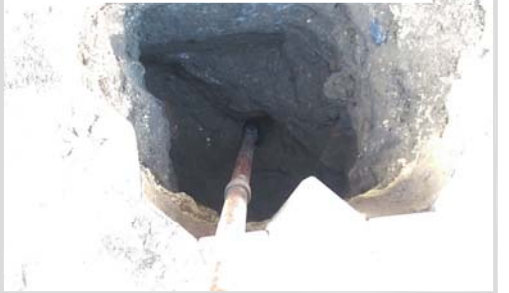
VIEW: PROBING WORKS TO DETERMINE THE BASE OF THE CONCRETE FOUNDATION AT THE UPPER LEVEL
