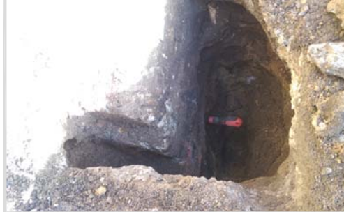
VIEW: EXPOSED CONCRETE FOUNDATION FROM GROUND LEVEL
