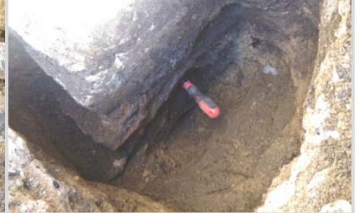
VIEW: SCREWDRIVER PLACED AT BASE OF FOUNDATION
